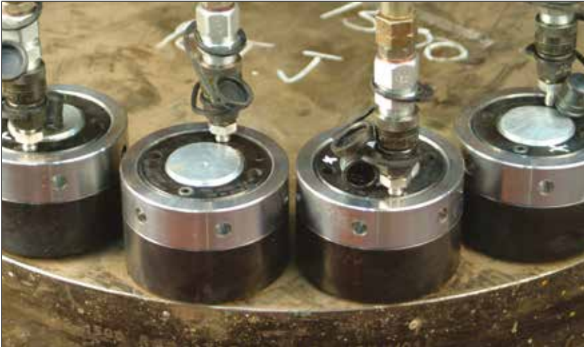
▲ Tensioning with hydraulic nuts.
