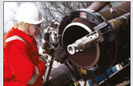
▲ Pipe cutters and weld preparation.
