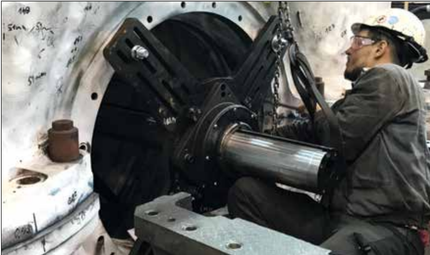
▲ Pipe cutters and weld preparation.
