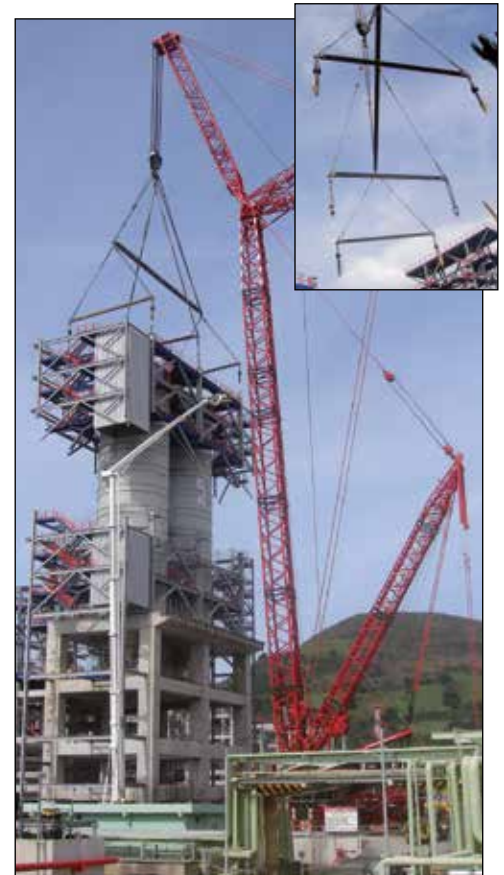
SyncHoist system mounted in an auxiliary frame for levelling and positioning steel structures during construction of an oil & gas installation. ▶
